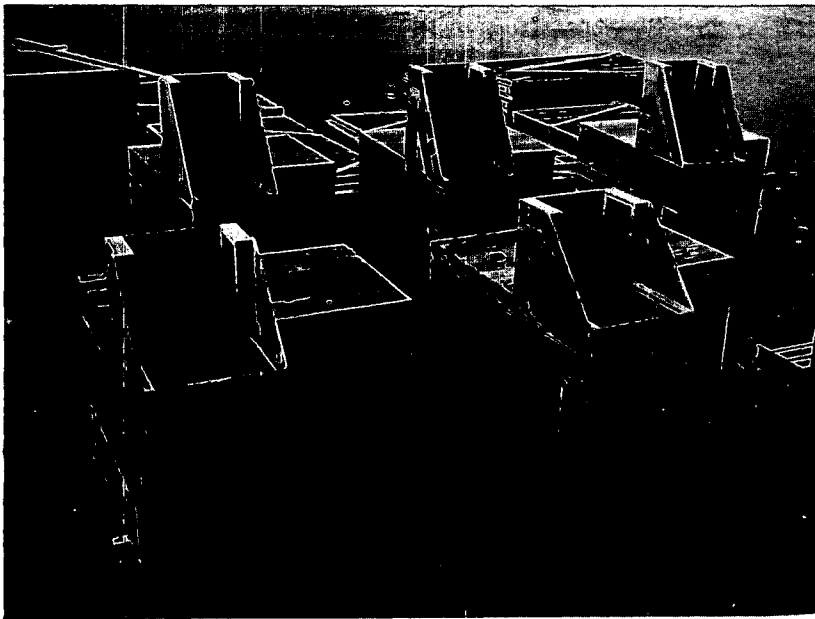
Fig. 1—Prefabricated structures for covered-trench shelters (carpentry yard).
